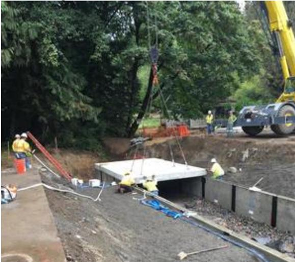
Installing culvert lid after fish rock installed at NW 8th Ave with team in culvert (1)
