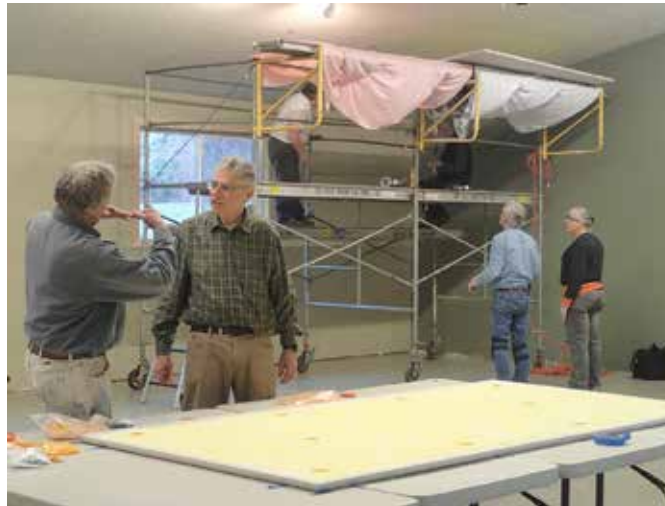
A hard-working crew of volunteers installing acoustical panels on the ceiling and walls of the Skyline Grange (Photo: Sen Speroff)
